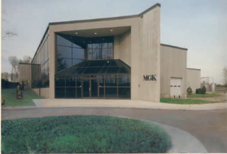
The Chaska production plant
